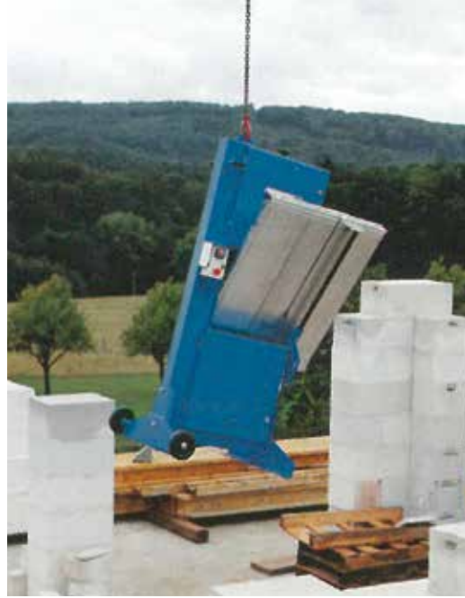
Gut erreichbare Transportöse Accessible transport lug
